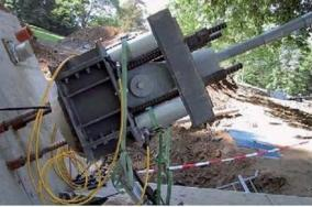
Figure 42: Foundation Cable Tensioning Device, Tensile Surface Structures, p. 103
